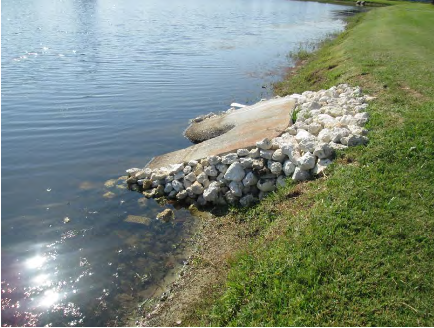
MES Repair on west side of Pond 7
