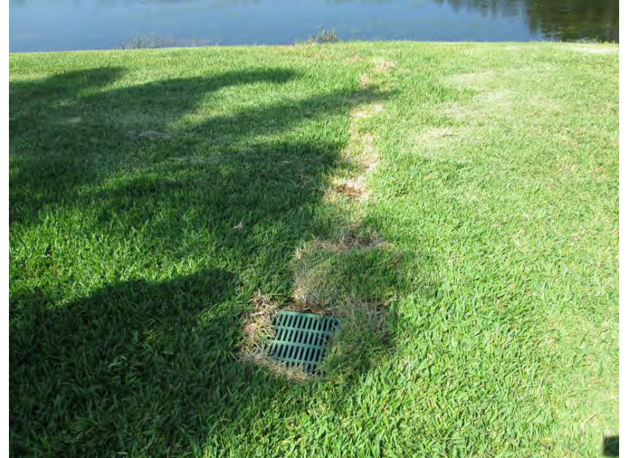
New grate at northeast side of Pond 16 needs edging – punch list item
