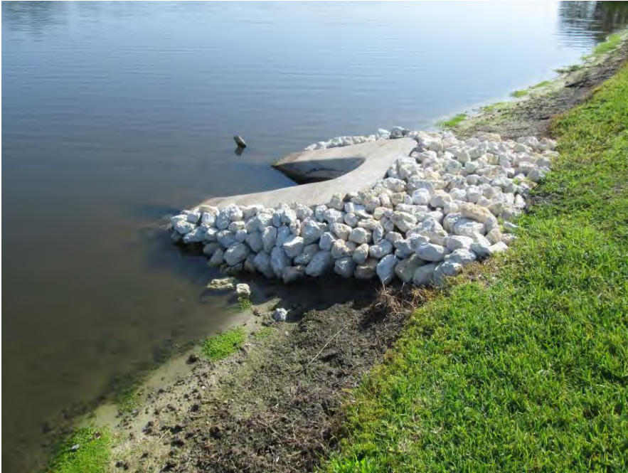
MES repair near southwest corner of Pond 9
