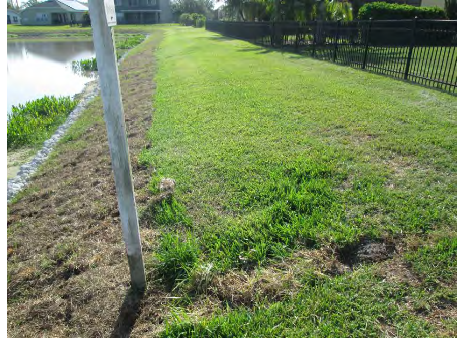
Depression on south side of Pond 8 – punch list item
