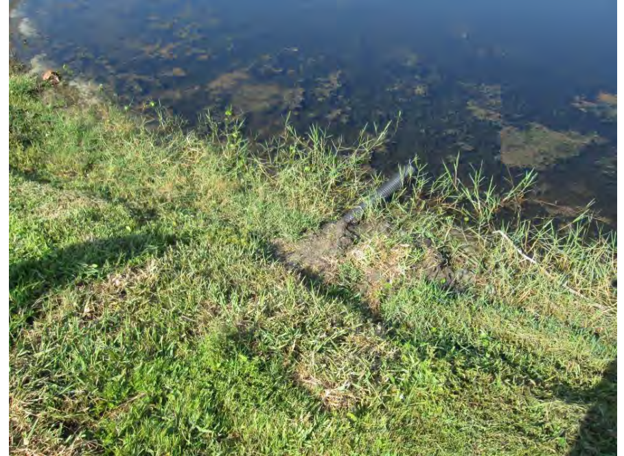
Spot Repair at southeast corner of Pond 7 needs rip rap – punch list item
