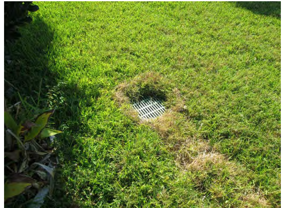
New grate at southeast corner of Pond 7 needs edging – punch list item
