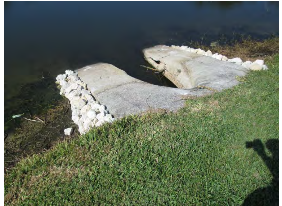
MES Repair on northwest side of FCA-2
