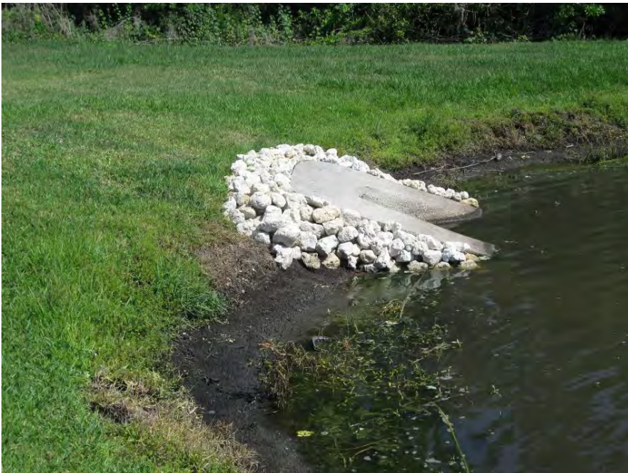
MES Repair on northwest corner of Pond 2
