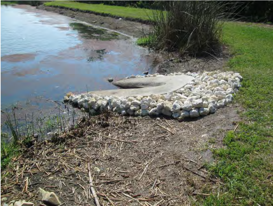
MES Repair on southwest side of Pond 11
