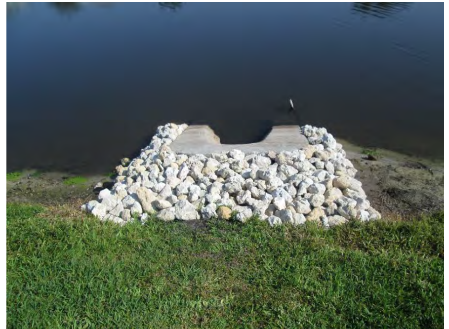
MES repair near southwest corner of Pond 9
