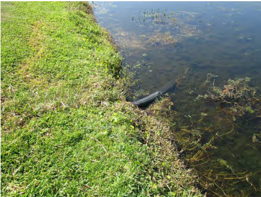
Spot Repair at northeast side of Pond 16 needs rip rap – punch list item
