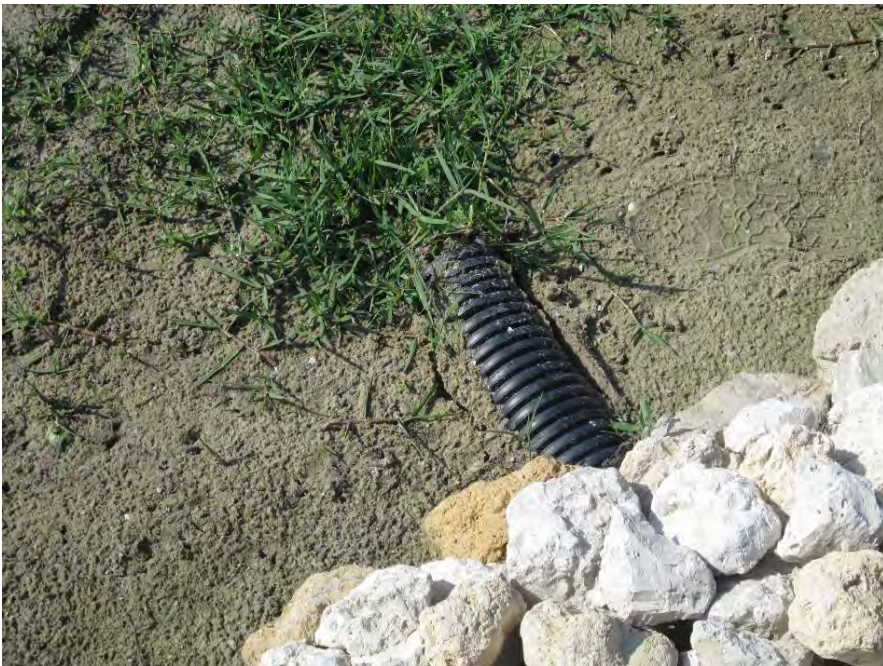
Drainage pipe partially buried – punch list item
